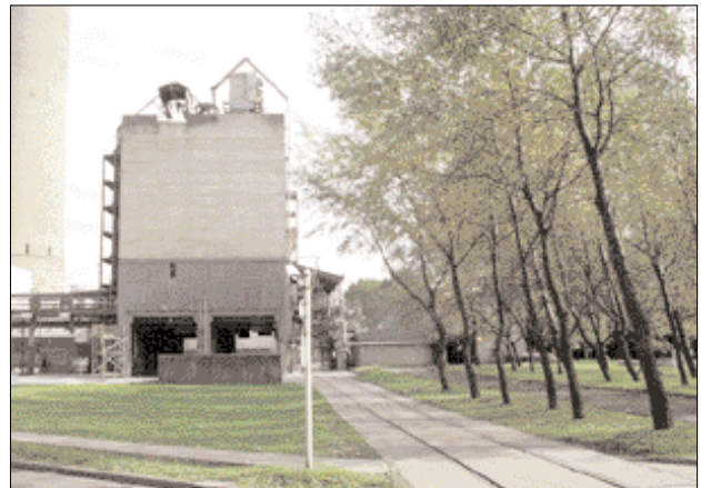
Figure 3. Dry pulverised fuel ash storage silo at Didcot Power Station (courtesy of Innogy plc)
