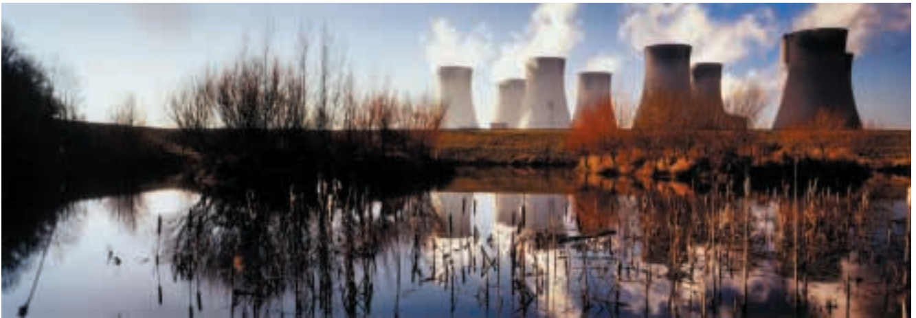
Figure 13. Coal-fired power station (courtesy of Powergen)
