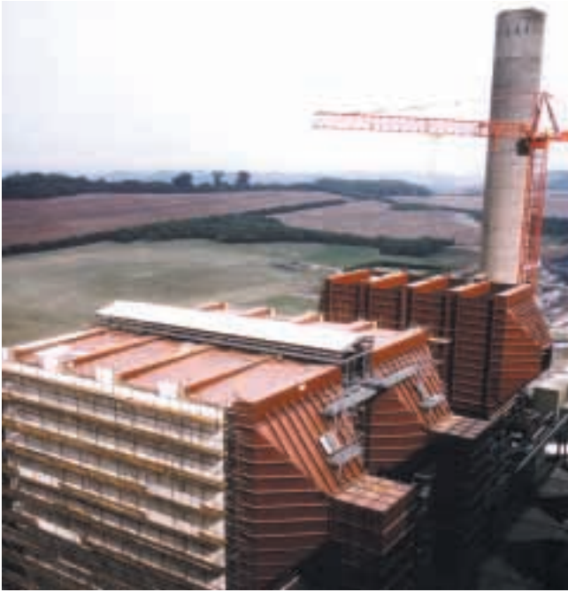
Figure 9. Electrostatic precipitator refurbishment (courtesy of Powergen)
