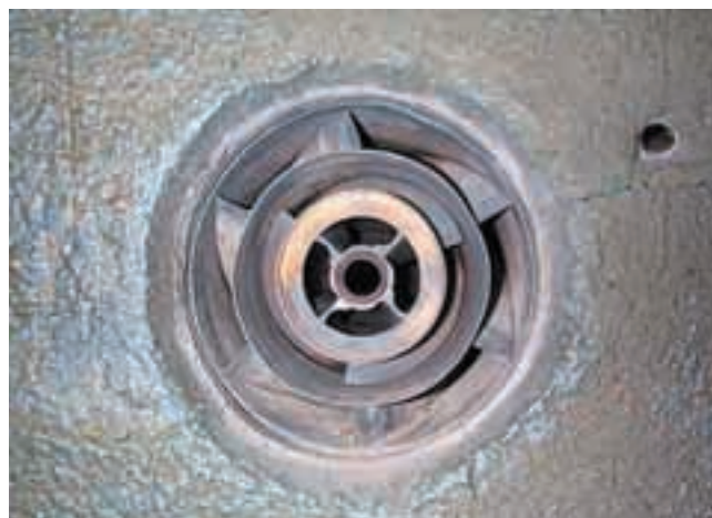
Figure 8. Low-NO x burner (courtesy of Powergen)
