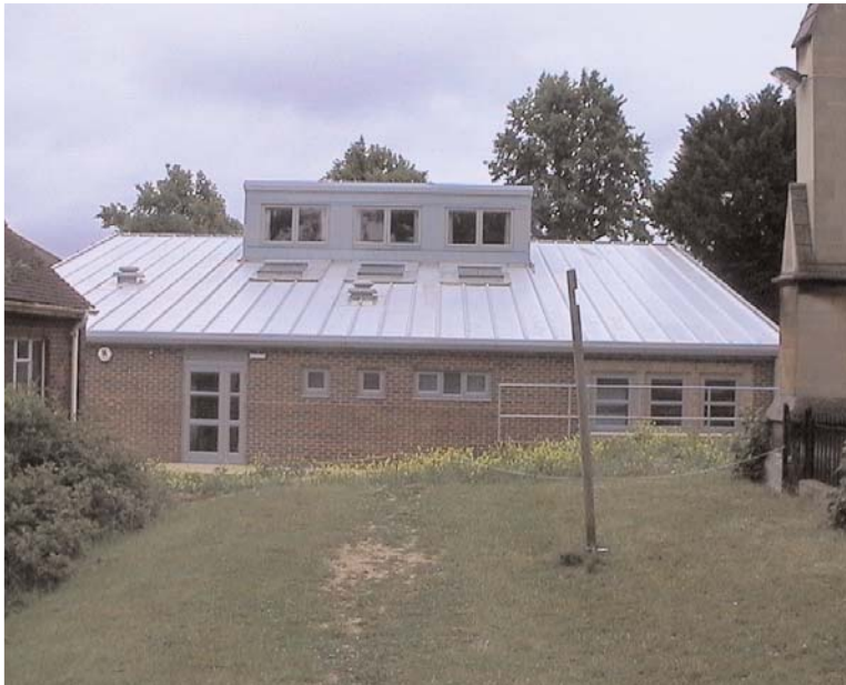
Left: The north side of the building has high level windows to allow daylight without overheating in summer. Below: A high ceiling and lots of light make the new church hall airy and attractive.
