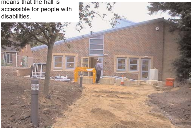
Above: Glazing is modestly proportioned to prevent big thermal losses in winter.
